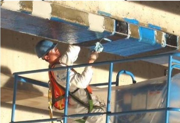
Figure 1: A Typical FRP Strengthening Process of bridge deck
