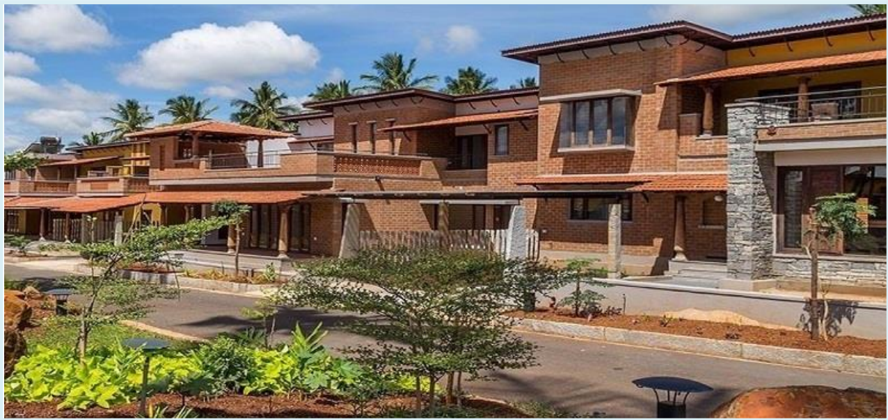
Fig. 1. T-Zed Homes at Old Airport-Whitefield Road, Bengaluru
