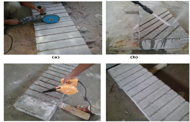
Figure (2) Grooves Preparation on Beam Side Face
