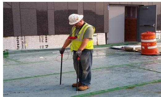
Fig.2. EFVM testing for leakage in roof
