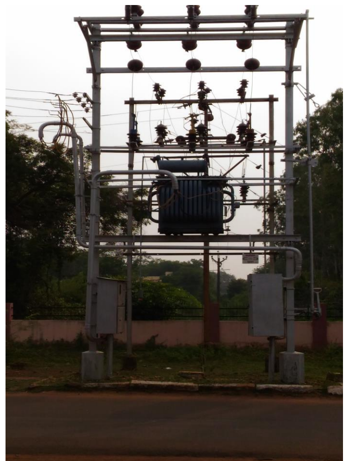
Fig. 1. View of the deteriorated electrical substructure (a) elevation view of the full structure; (b) U-clamp connection (bolted): sectional view; (c) U-clamp connection (bolted): back view; (d) flange-to-flange bolted connection
