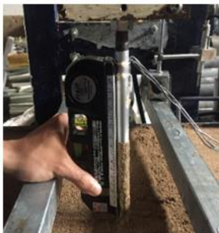
Figure 5. Pile lowering process – Check the verticality and press
