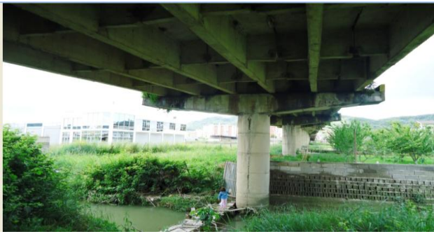
Fig. 2. Overview of girders superstructure
