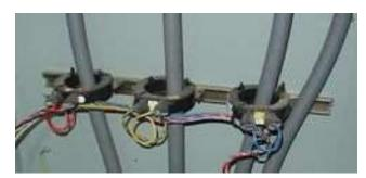
Current transformers used in metering equipment for threephase 400 ampere electricity supply
