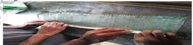
Fig. 1 Wrapping steel bar with epoxy coated glass fibre fabric
