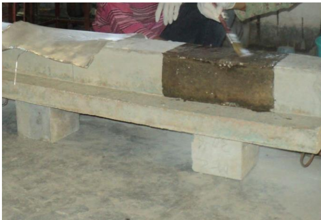
Fixing of FRP sheets on the beam
