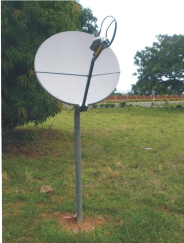
Fig 8. Outdoor Unit (ODU) of VSAT, CGG, Toro, Nigeria
