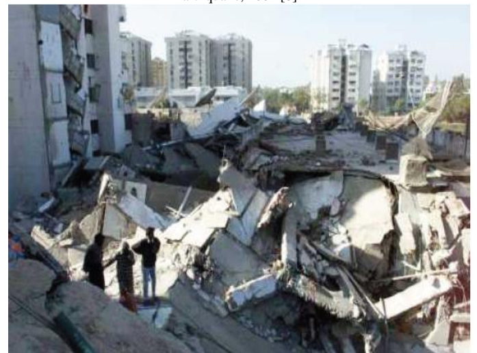
Figure 2: Collapse of 9 storey apartment buildings due to soft storey at Ahmedabad during Bhuj Earthquake, 2001 [8]
