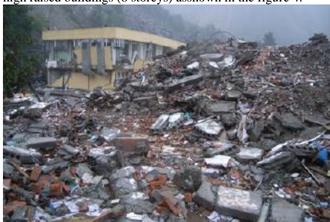
Figure 3: Collapse of school building due to effect of soft storey at Yingxiu Town of Wenchuan County during Wenchuan Earthquake, 2008 [2]
