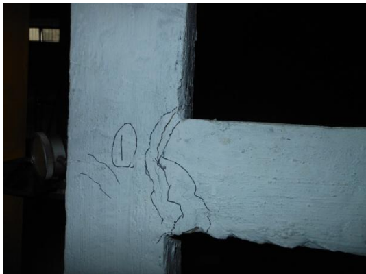
c. Far end of loading story 1
