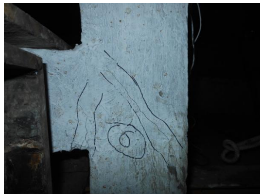
f. Near end of loading plinth level
