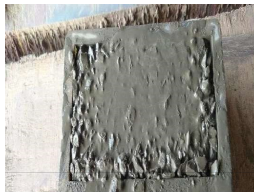
Fig.4. Casting of blocks
