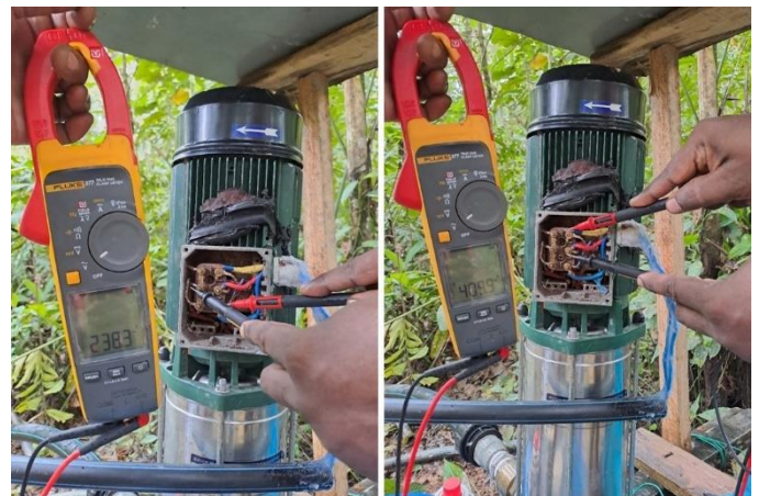
Fig. 8: The phase to star point voltage is V=238V and the \Phi - \Phi voltage is 409.9V.
