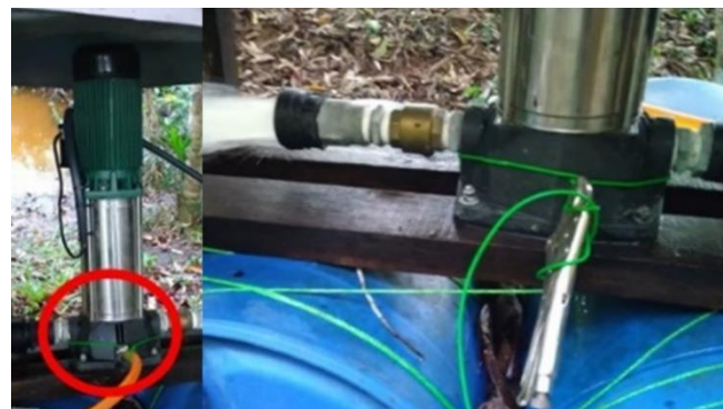
Fig. 1: Priming the 4 HP pump
