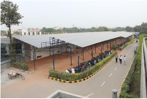
Fig.2. Schematic view of PV system installed in the North Cap University, gurgaon, India.
