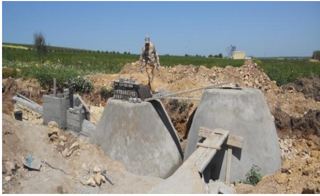
Figure 2. Construction of digester by dome in the region of Khouribga
