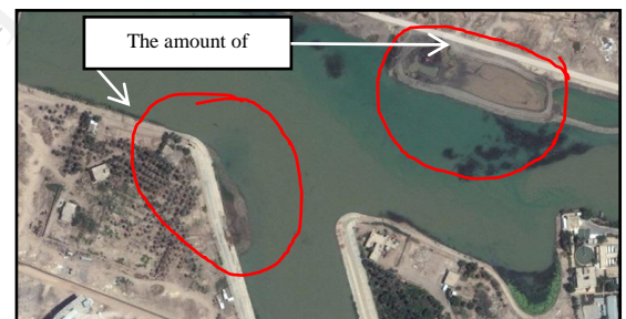
Fig. 10: The Location of Sediment Accumulation in the Right Bank at Branch to Barrage. (Google Image, at 2013)
