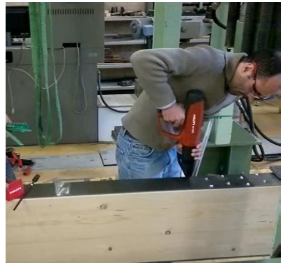
Figure 3: Reinforcement with thin steel plates on both sides connected with driven nails
