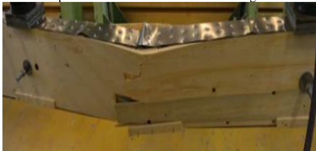
Figure 12: Failure pattern under ultimate load C1-CLT-N
