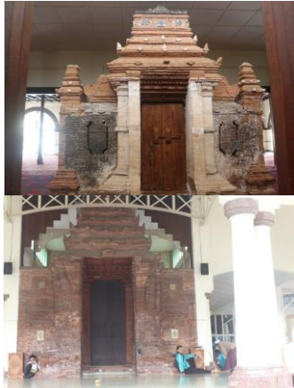
Fig. 20. Kembar Gates which are in the Mosque's Porch and Inside the Al-Aqsa Mosque Kudus
