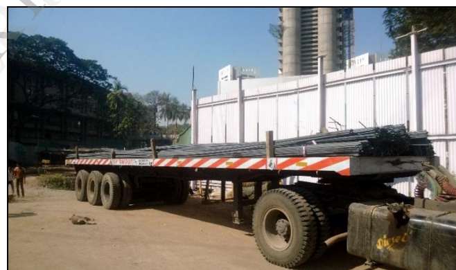
Fig. 2 Steel Received at the steel yard
