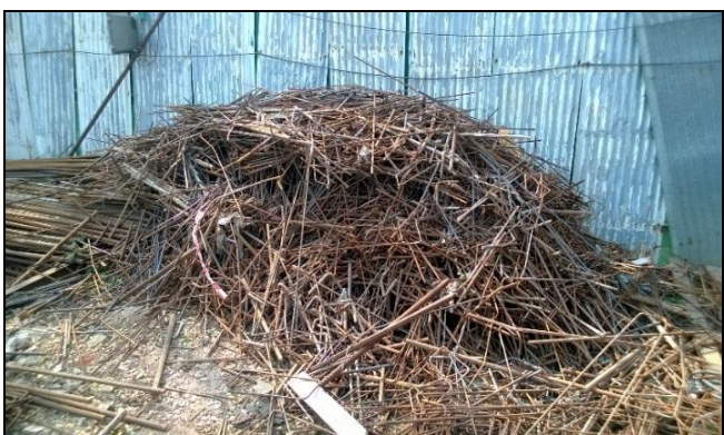
Fig. 5 Waste of cut pieces of steel
