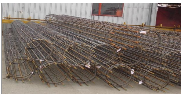
Fig 11. Off-site fixed column cages
