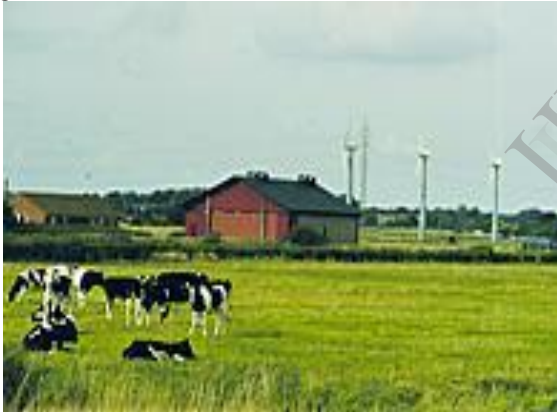
Figure 4.5 H Tjaereborg VSC Light converter station [16]
