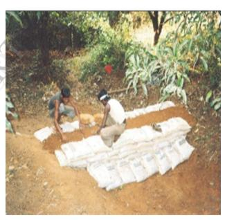
Vanrai bandhara are constructed just after the last rains to arrest the runoff and store water .For few months into the dry season. The typical height of a vanrai bandhara is about 0.8 m to 1.2 m. Length of the bandhara ranges from 6-7 m up to 25 m. The breadth of the bandhara is about 2 m to 2.5 m. The bags used for the vanrai bandhara are 40cm x 30cm x 15cm (1 x b x h).
